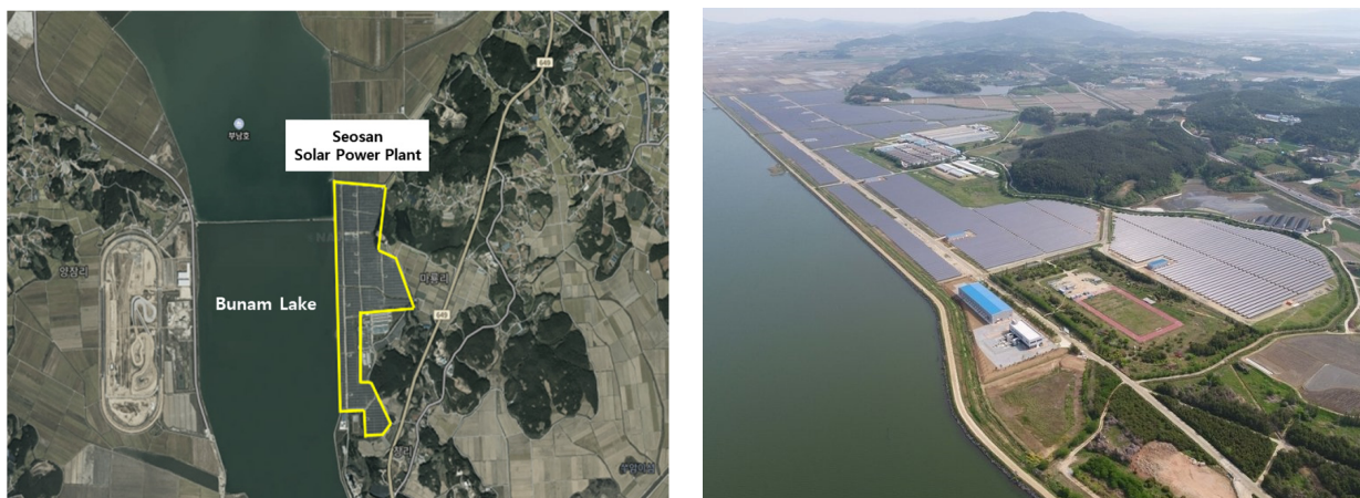
Figure 1. (left) Satellite image and (right) panoramic view of Seosan Solar Power Plant.
